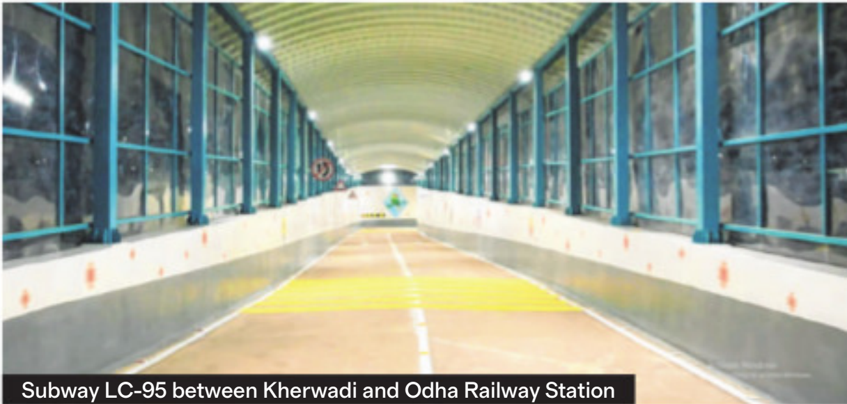
Subway LC-95 between Kherwadi and Odha Railway Station
