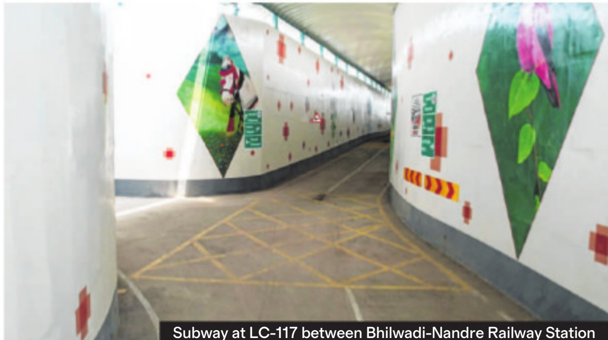
Subway at LC-117 between Bhilwadi-Nandre Railway Station
