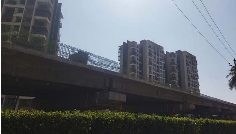
Construction of a ROB going on at Titwala |
