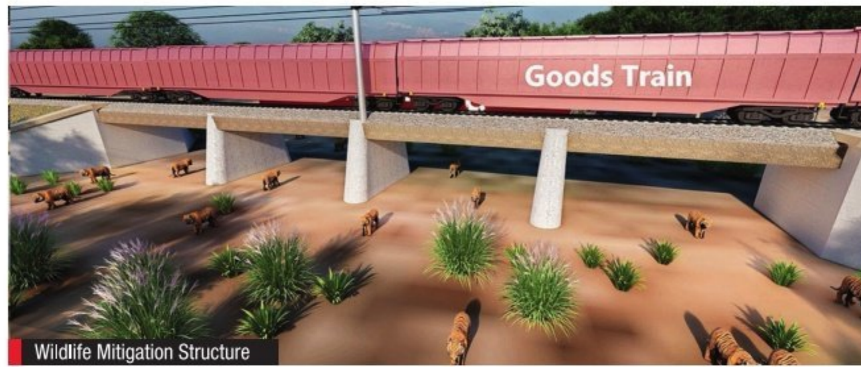
Wildlife Mitigation Structure
