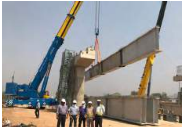
(b) Photo: Lifting of girder with lifting hook
