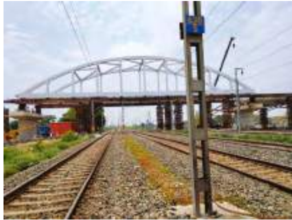
(g) Photo: Bringing BSG to its final location over piers
