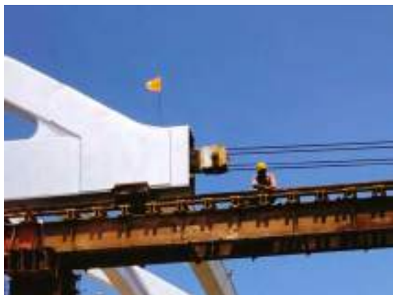
(e) Photo: Fixing Winch and rope assemblies
