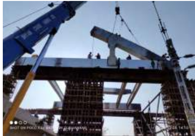
(b) Photo : Start of assembly of Bottom Beam, Top Chord, Hangers and Cross Girders
