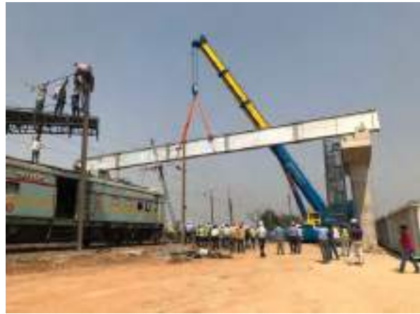
(d) Photo: Crossing of girder across track
