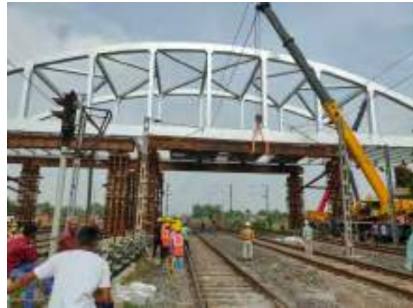
(b) Supporting of BSG over piers and removal of beams
