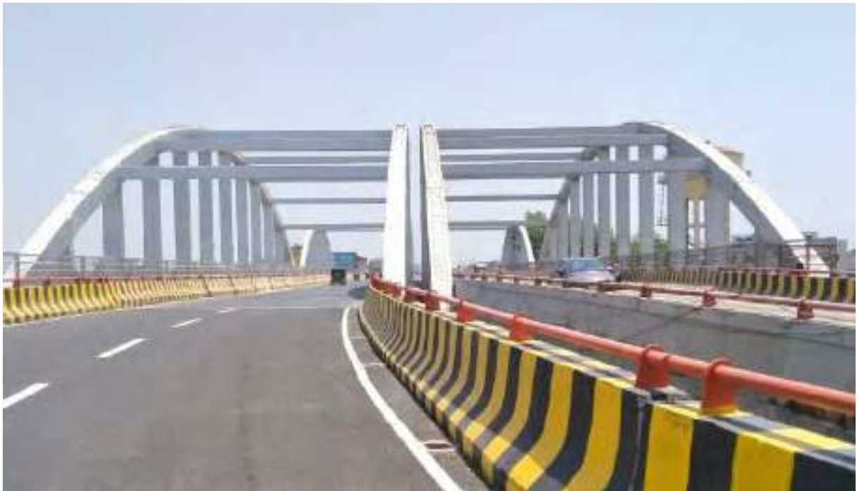
Fig. c): Bow String Arch Steel Girder
