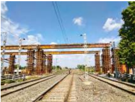
(c) Fixing longitudinal beams and Trestles
