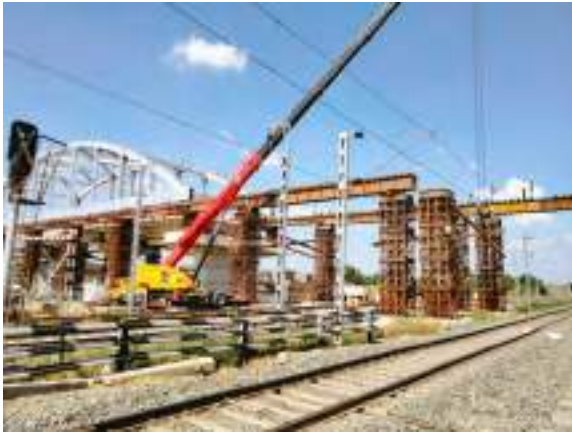
(a) Photo: Erection of temporary arrangements- Trestles
