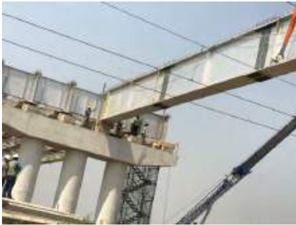
(e) Photo: Placing of girder in position
