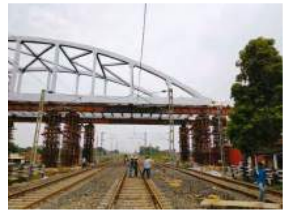
(f) Photo: Launching of BSG over temporary arrangements
