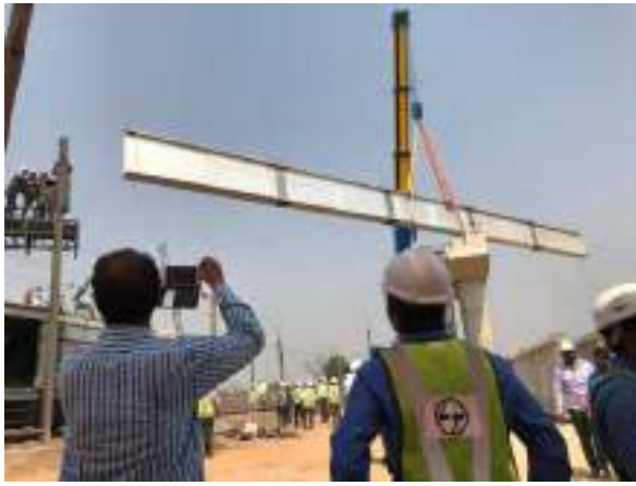
(c) Photo: Lifting of girder
