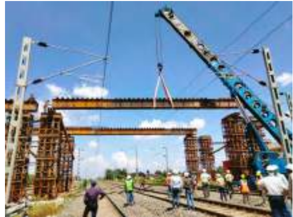
(b) Photo: Erection of temporary arrangements- Longitudinal Beams
