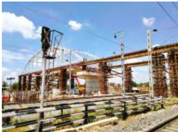
(d) Photo: Completing Temporary arrangements for launching
