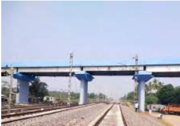
Fig. a): Composite Steel Plate Girder
