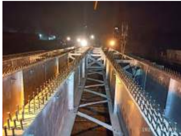
(f) Photo: Placing of all girders in position, secured in place
