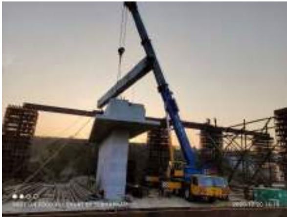
(a) Photo: Erecting temporary arrangements
