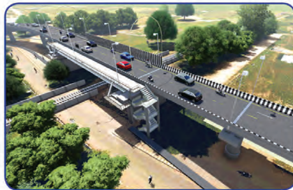
LC 34 : ROB at Wardha- Ballharshah between Manjri - Bhandak station
