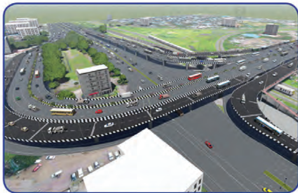
Widening of Turbhe ROB
