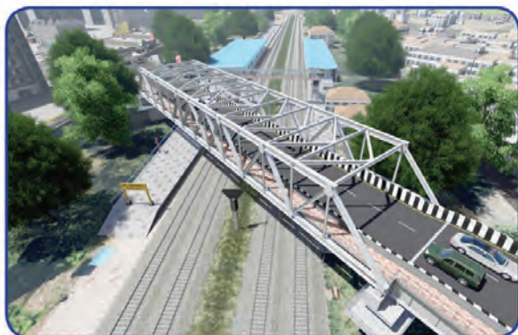
LC 112 : ROB at Pune-Miraj Near Kirloskarwadi Yard
