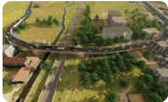
Road Over Bridge (ROB) at LC 116 at Gumgaon on Warha - Nagpur section on Central Railway in Nagpur district
