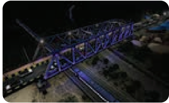
Road Over Bridge (ROB) at LC 43A-143 in Babupeth near Chanda Fort Rly. Station in Chandrapur district
