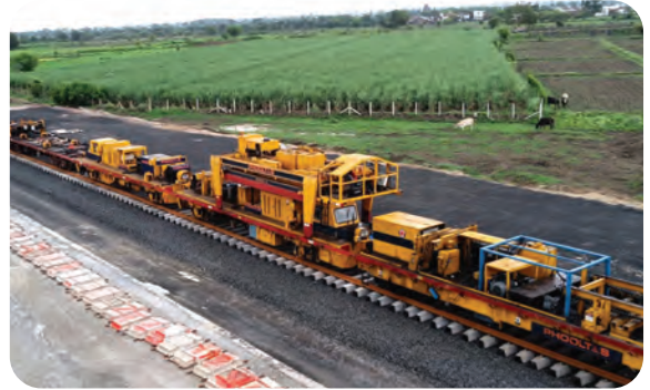
Laying of Railway track by New Track Construction (NTC) machine for Nagpur (Itwari) - Nagbhid GC project
