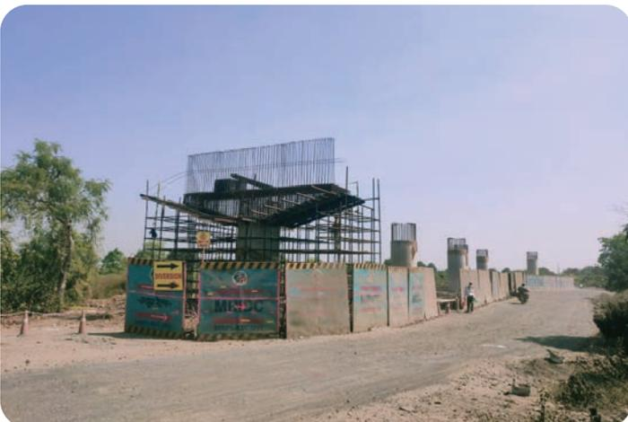
LC 290: Fixing of Reinforcement for Pier Cap
