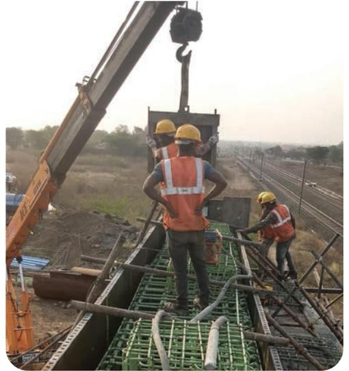
LC 136: Concreting for Pier cap
