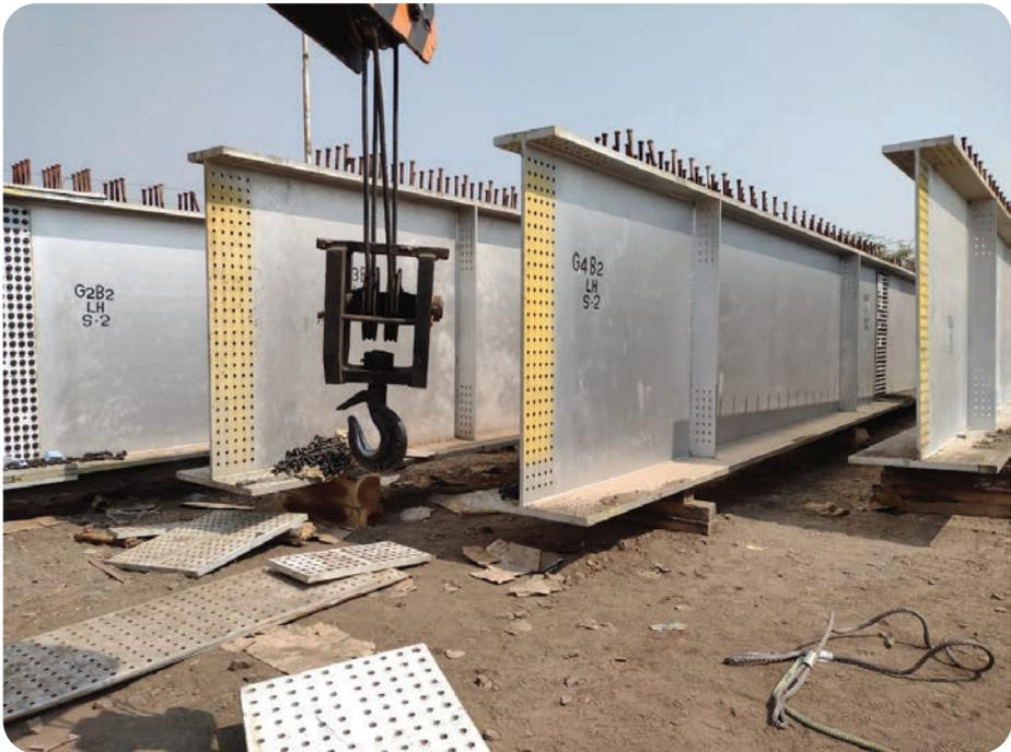
LC 112A: Railway Span Steel Girder Assembly work
