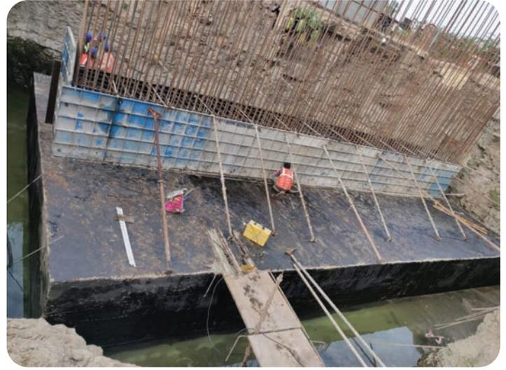
LC 134A: Fixing of reinforcement for open foundation
