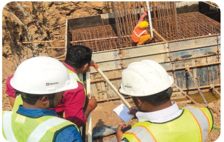
LC 20: Level Checking of Pier and Pier Cap
