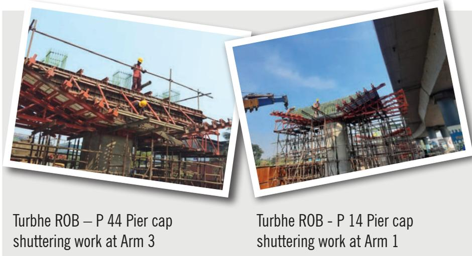
Turbhe ROB – P 44 Pier cap shuttering work at Arm 3
