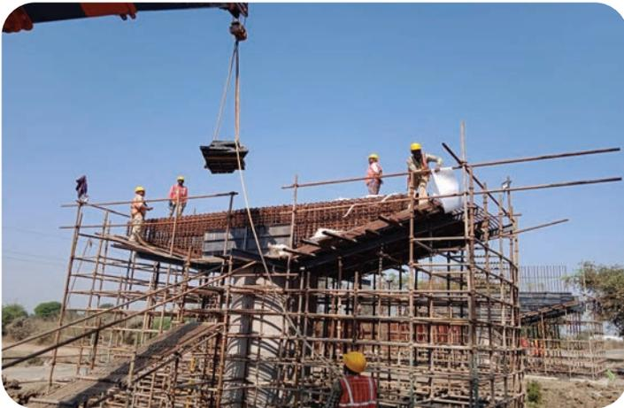
LC 290B: P1 Pier Cap shuttering work
