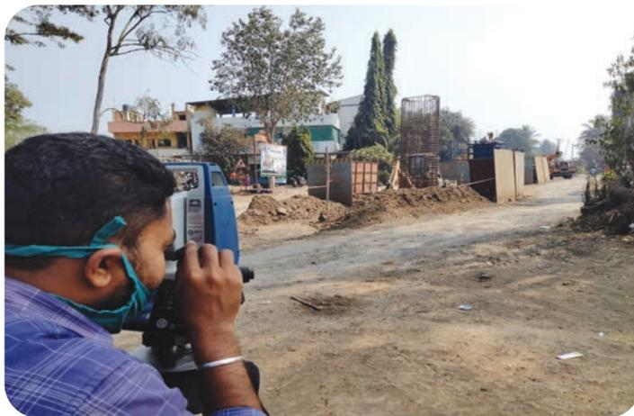
LC 81: Pier level checking work
