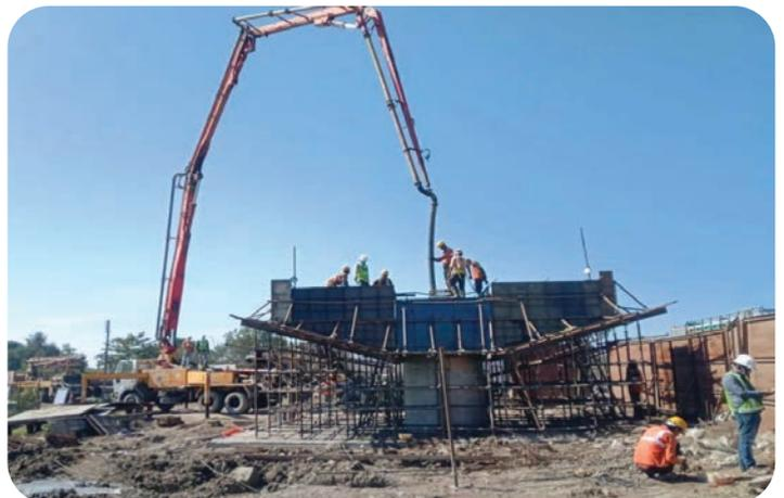
LC 103: Concreting of Pier
